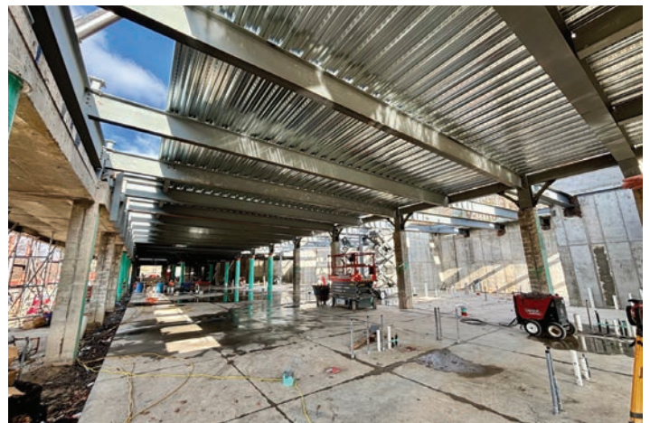
Ceiling of the first floor nearing completion.
